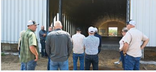
New storage under construction at the Offutt Farm near Park Rapids.
